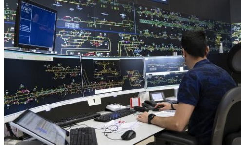
CBTC SIGNALLING SYSTEM FOR HELSINKI (FINLAND)
